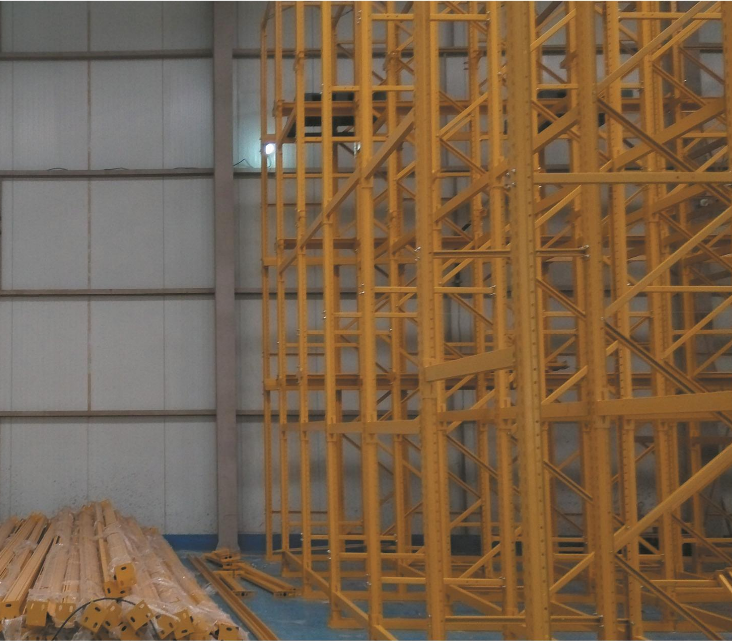
BIOPACK Company Warehouse Drive-in Rack System Project(2015).
